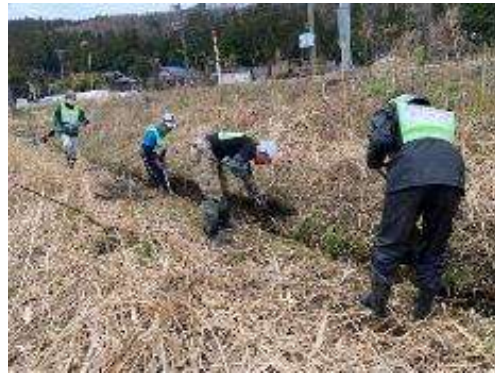
Mud lifting in waterways (Wajima City, April 3)
